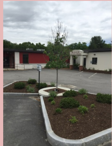
Image of a tree box filter installed at the Wiggin Memorial Library in Stratham, NH that will capture silt, oil, nitrogen, and other pollutants from rain runoff. (Source: SRPC)
